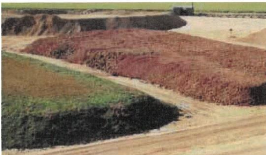
Clearly defined stockpiling of different soil materials
