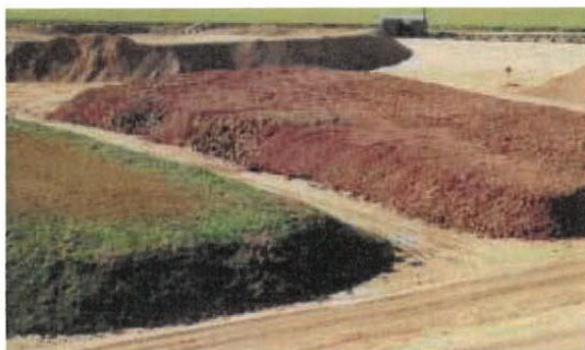
Clearly defined stockpiling of different soil materials
